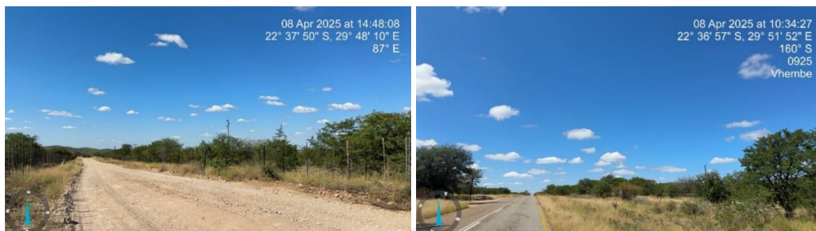
Photo 7.39: Overhead power lines protruding above the tree line
