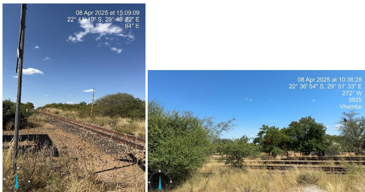
Photo 7.32: Existing railway line
